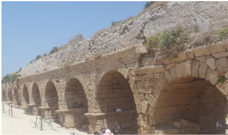
Aquaduct in Caesarea
